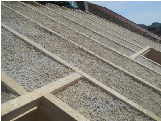
INSULATION OF ROOF
