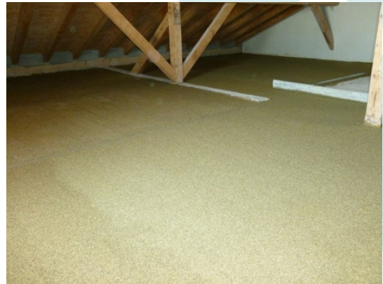
INSULATION OF AN ATTIC
