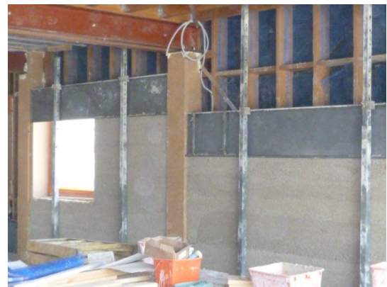
HES-mix MOUNTED WITH FORMWORK
