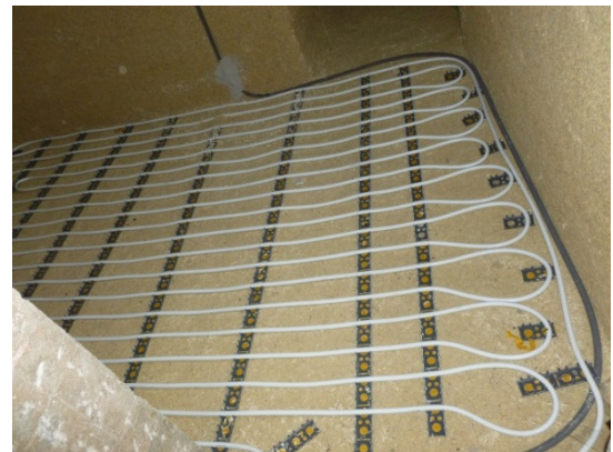
HES-mix WITH FLOOR HEATING
