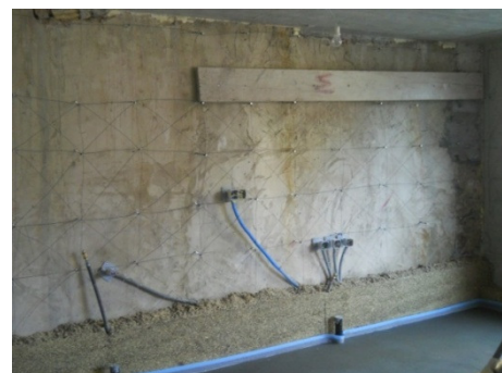
TUBING INCORPORATED IN HES-mix
